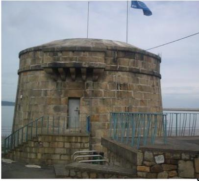
The Martello door was placed up high, facing the land and entry for the soldiers was by ladder. Above the entrance door there was a slotted platform or grill called a machicolation which allowed for downward fire on attackers.
